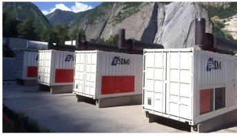
Pic. 2. The four 1900 kVA generating sets installed at the foot of the Pas-du-Roc cliff
