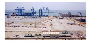
View of the outside of the backup power plant in the foreground with two fuel tanks (left), and the building housing the four generating sets (center)
