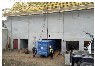
Pic. 2: Installation of the 550 kVA generating set in the specially constructed  $27m^2$  equipment room
