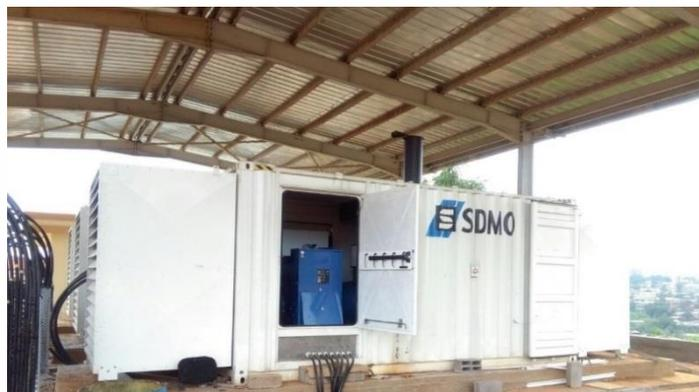
*Pic. 1. Three generating set individually installed in three Super Silent Containers.*
